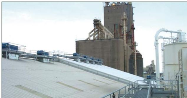
Figure 2. By distributing the dust collectors across the roof of the Southern Cement warehouse, the air in the entire building is efficiently changed every hour, which improves visibility and working conditions.
