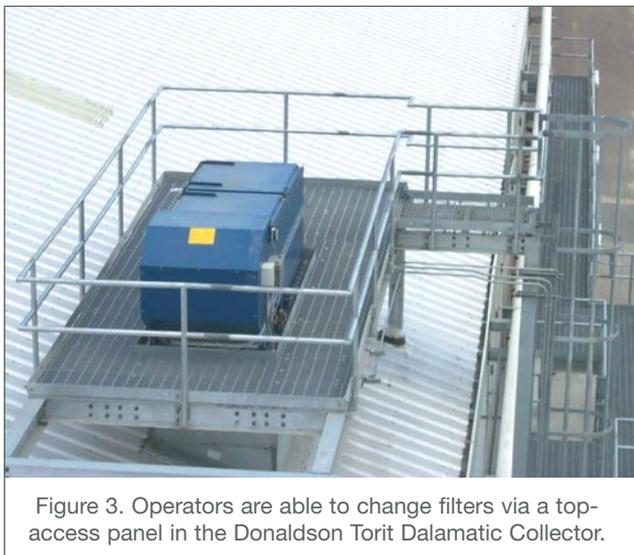
Figure 3. Operators are able to change filters via a top-access panel in the Donaldson Torit Dalamatric Collector.
